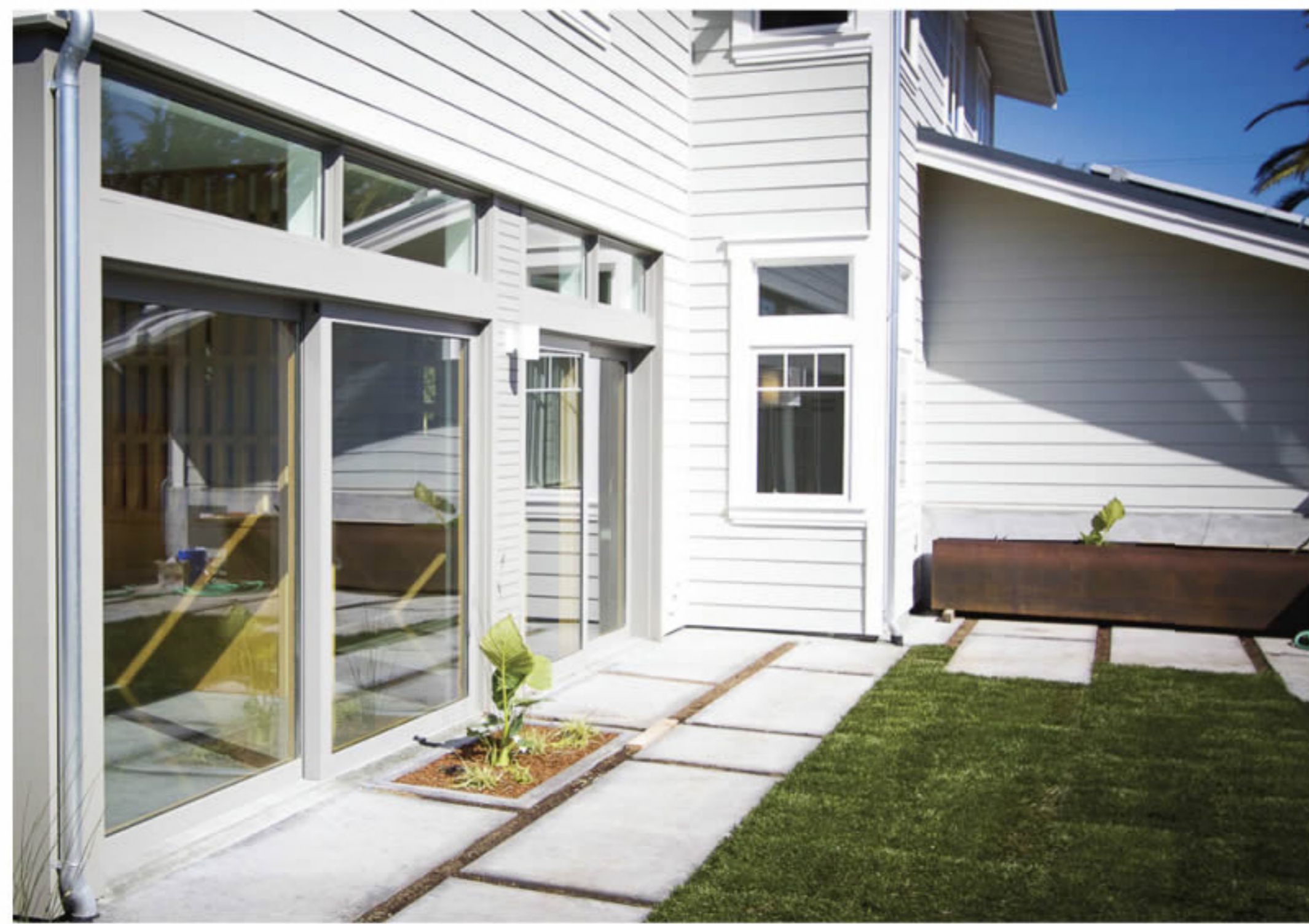
The home's exterior siding is a cementitious fiber board which has high fire resistance, moisture and rot resistance and a longer cycle time between painting.
